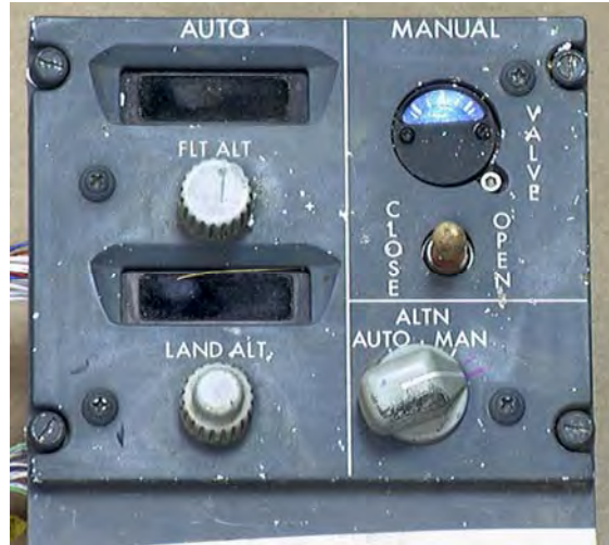
Photo – Pressurization Panel
