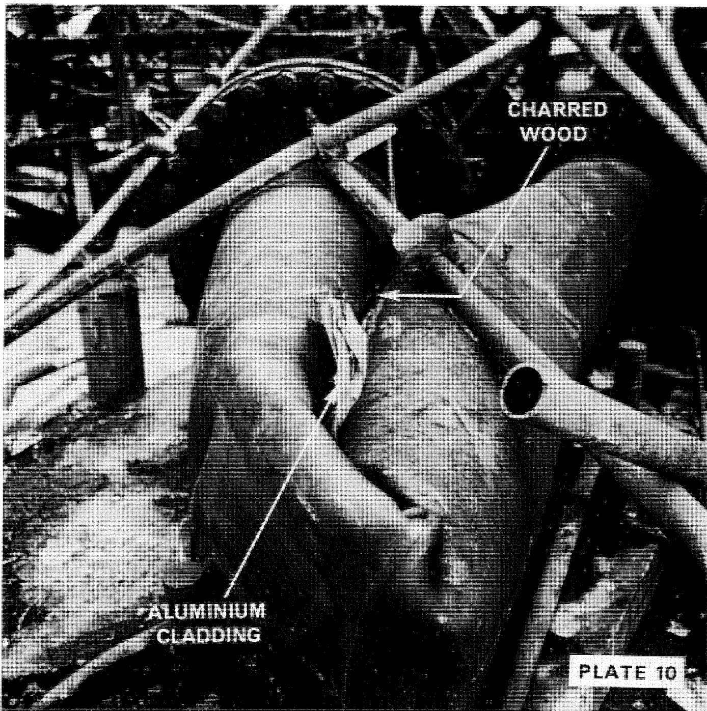
Plate 10 The jack-knifed 20 inch pipe showing trapped aluminium cladding and charred wood.
